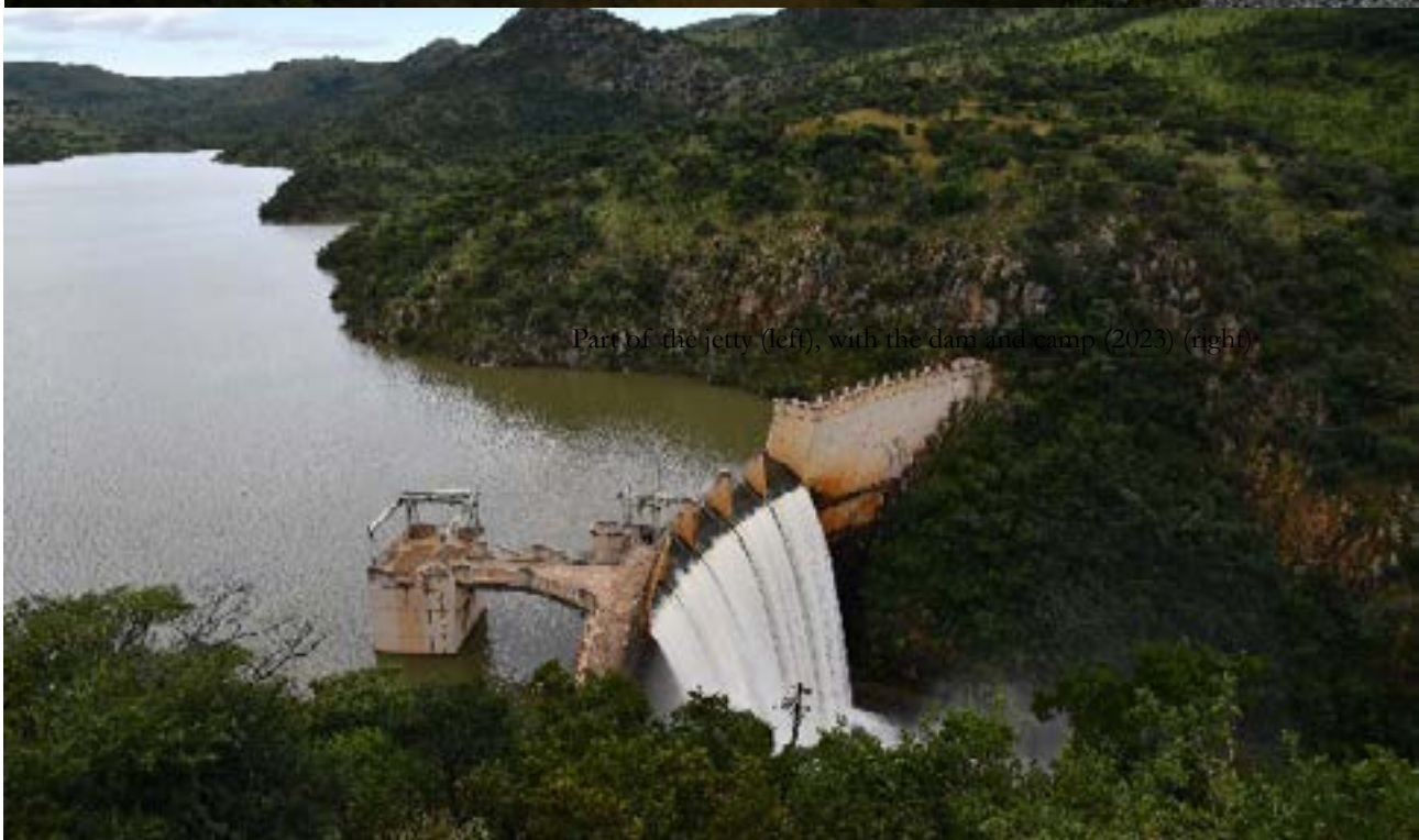
Bivane Dam in 2023 (overflowing) (top), versus 2015 (bottom)
